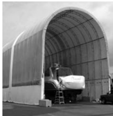
The new portable shelter is 30’ by 100’.
